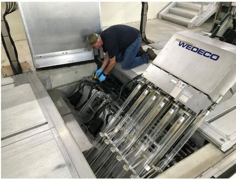
Instrument technician testing position switch. 9/13/2021
